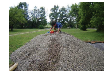
THE BUILDING GROUND PILES OF RAW MATERIAL
